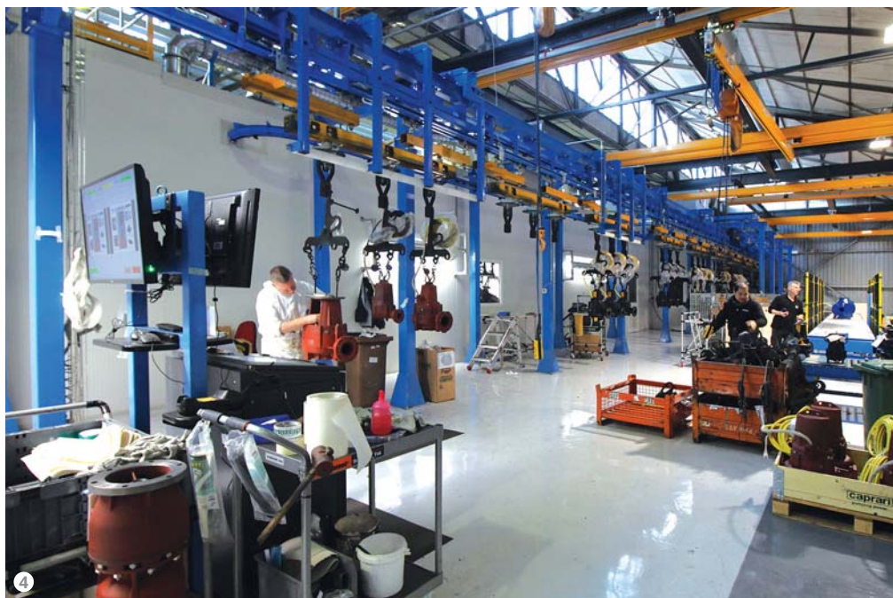
Figure 4: A part of the new coating plant installed by Trasmetal (Milan).
